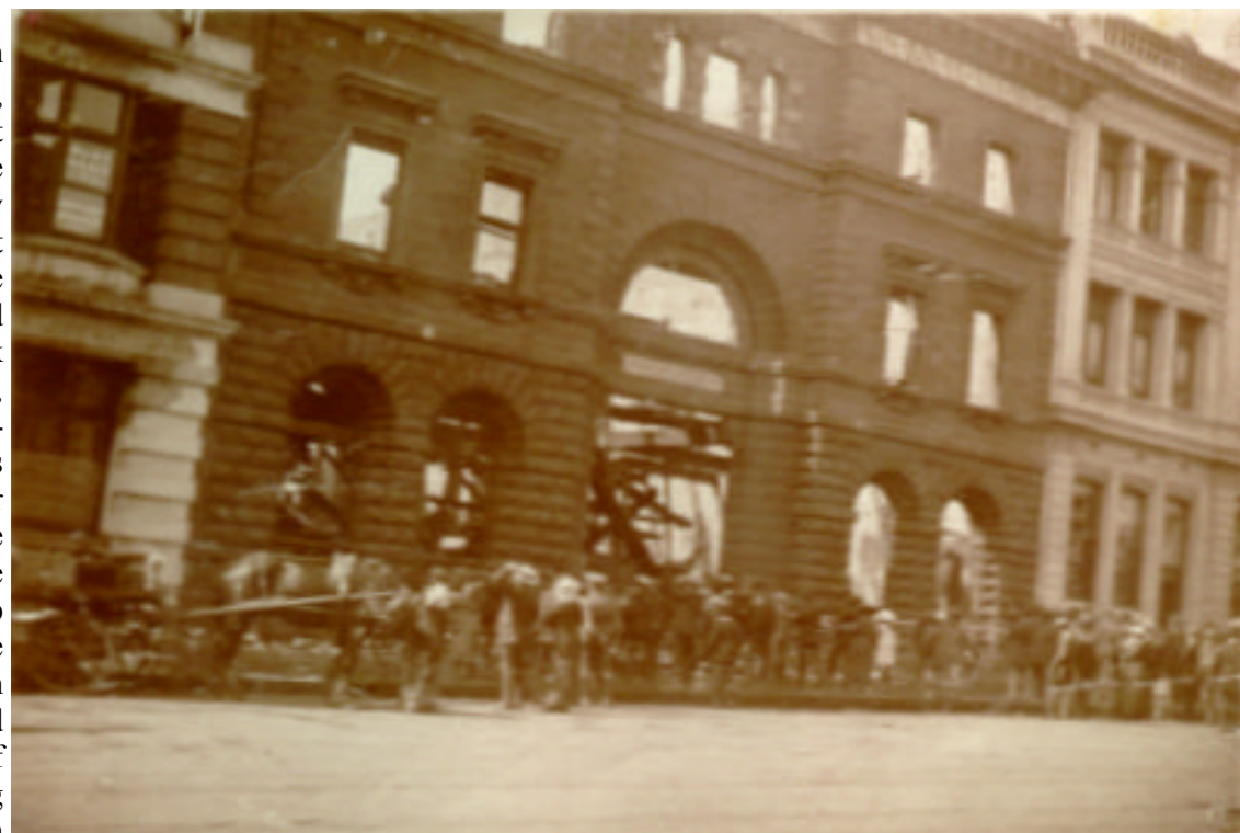
Above: This burnt-out shell is all that remained of the once grand blue-stone building occupied by the printing firm of Andrew Jack, Dyson & Co.
