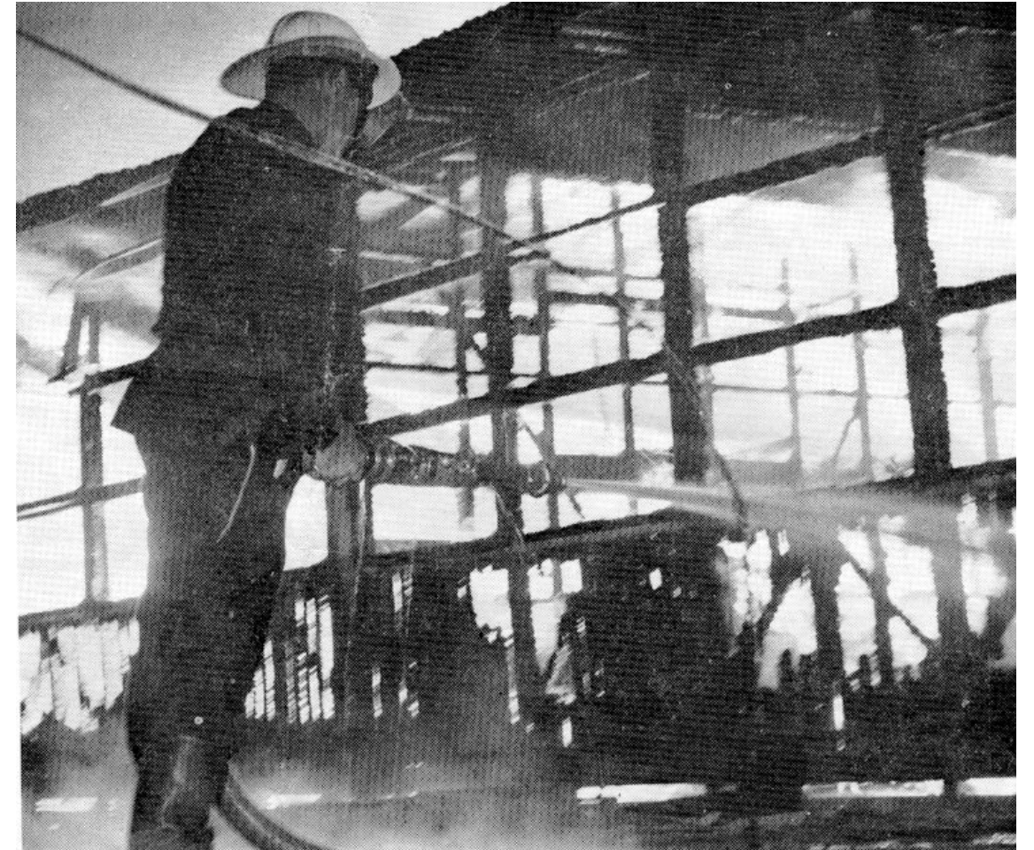
Fire destroyed these classrooms and a craft room in the infants section of the Heidelberg State School, Victoria.
