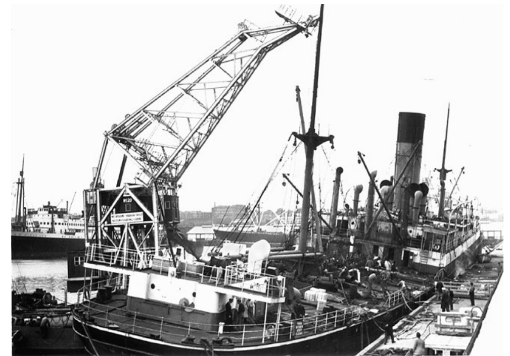
Above: The Harbour Trust's giant floating crane, the largest of its type in the Southern Hemisphere, placed a number of high pressure pumps on board the stricken ship, in readiness for the refloating attempt.
