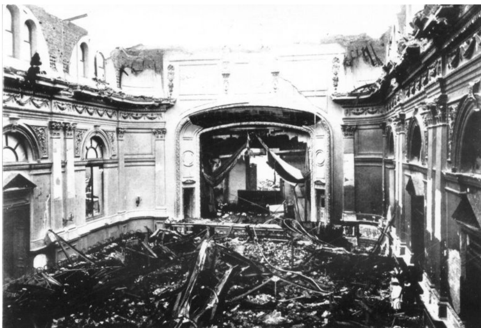
The gutted remains of the new portion of the Prahran Town Hall - the “City Hall”, as it was called.
