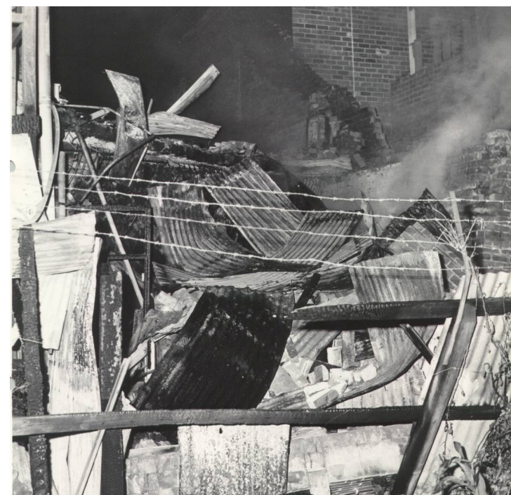
Above: Rear of the shop showing fence and barbed wire the Torch was propelled over by the force of the explosion.
