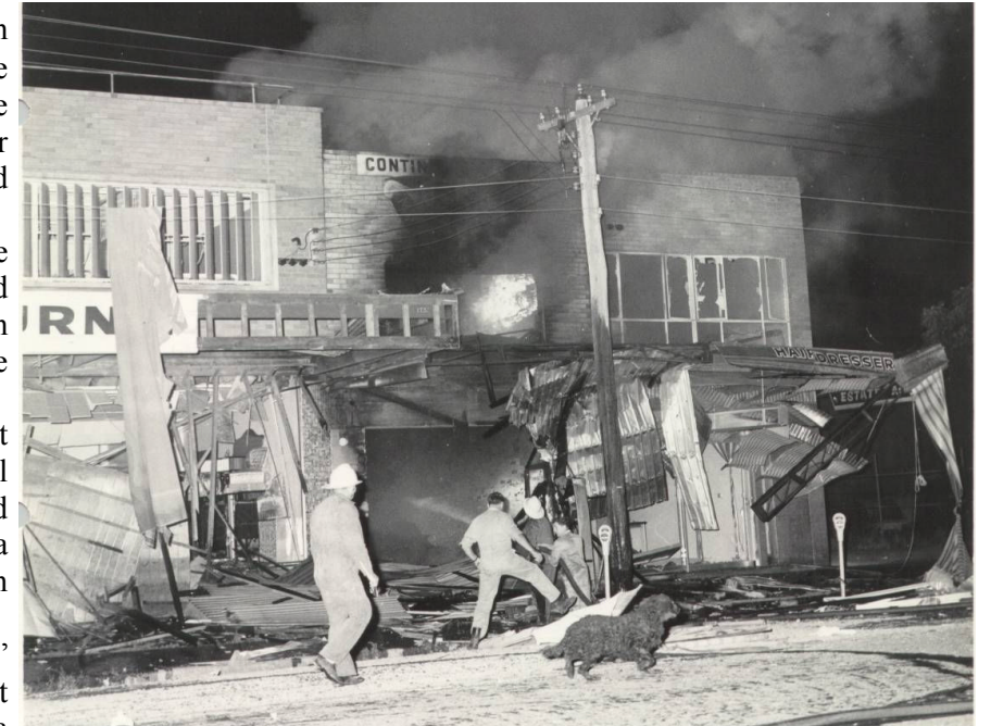
Above: Front view of the shop. Extensive damage to the surrounding shops led to their demolition. Thirty eight other premises incurred damage.
