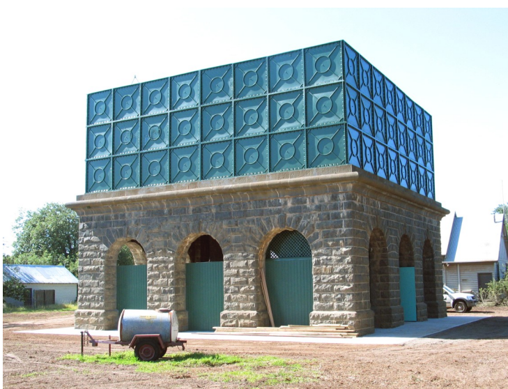
The water tank which was located on the Eye & Ear Hospital site opposite FS 1 at Eastern Hill. It was removed piece by piece from there to the Werribee sewerage facility. It has now been restored and is on public view.
