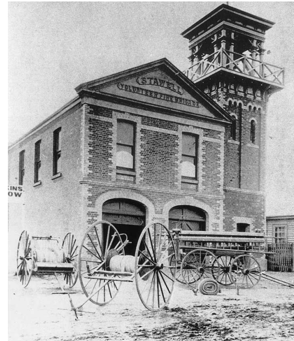
Hose reels and ladder outside the Stawell Volunteer Fire Brigade station circa 1890. A permanent water supply led to the universal use of hose reels.
